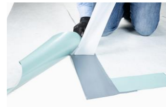
Sealing by butyl tape RENOLIT ALKORPRO BAND
