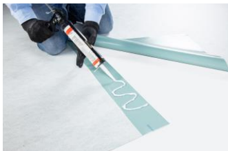
Sealing by mastic glue RENOLIT CEM 805
